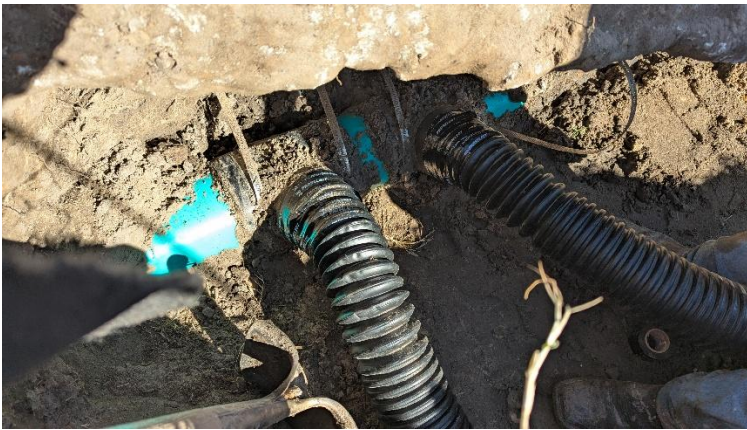
Figure 3 New solid cap added to underdrain stub on east side of structure. No damage present. Contractor wanted to put new cap to ensure proper seal.
