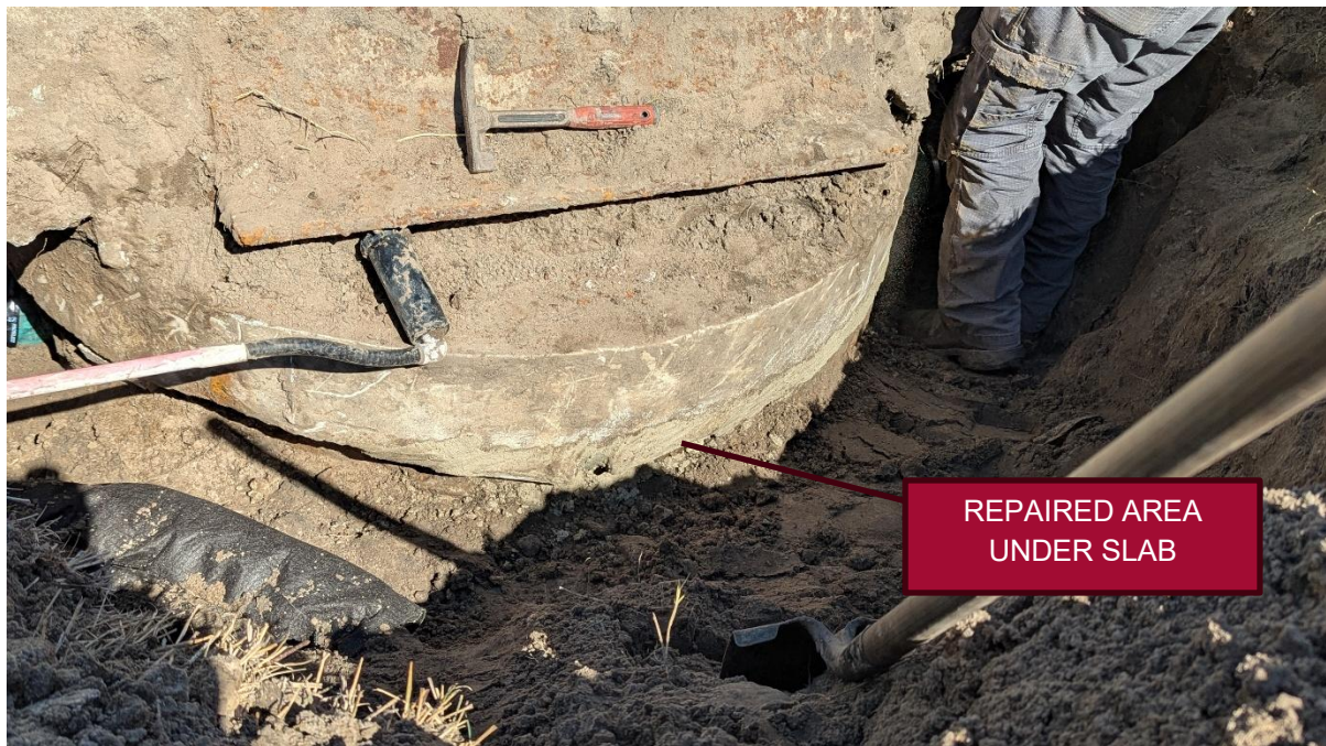
Figure 5 Completion of filling and mudding outside of structure at gap.
