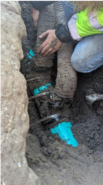
Figure 2 Photos of private drain pipes cracked from over bending when installed by DRH landscape contractor
