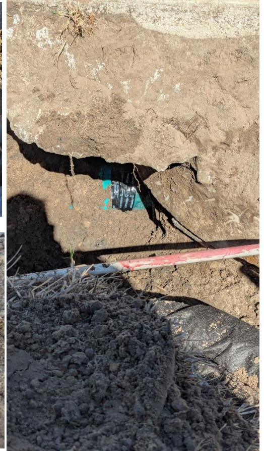
Figure 4 (Left) New solid wall plastic pipe installed to replace removed damaged pipe. All pipes pictured are part of private drainage system. Pipes and joints were subsequently wrapped in filter cloth as added layer of protection. (Right) Connection between underdrain stub (installed by Junior Davis as part of original construction) and the 6" solid green pipe (installed by DR Horton Landscape Contractor). Connection was excavated, examined, and additional sealing tap added to ensure solid connection.
