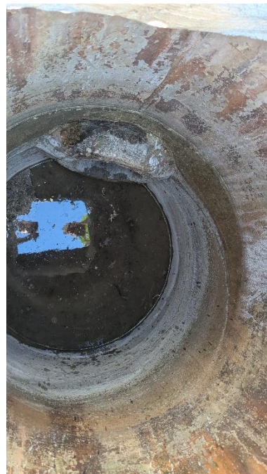
Figure 7 Image from inside structure where gap was repaired with waterproof mortar
