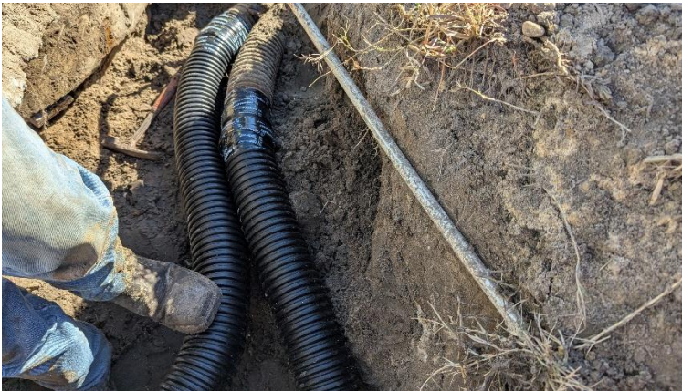
Figure 4 (Left) New solid wall plastic pipe installed to replace removed damaged pipe. All pipes pictured are part of private drainage system. Pipes and joints were subsequently wrapped in filter cloth as added layer of protection. (Right) Connection between underdrain stub (installed by Junior Davis as part of original construction) and the 6" solid green pipe (installed by DR Horton Landscape Contractor). Connection was excavated, examined, and additional sealing tap added to ensure solid connection.
