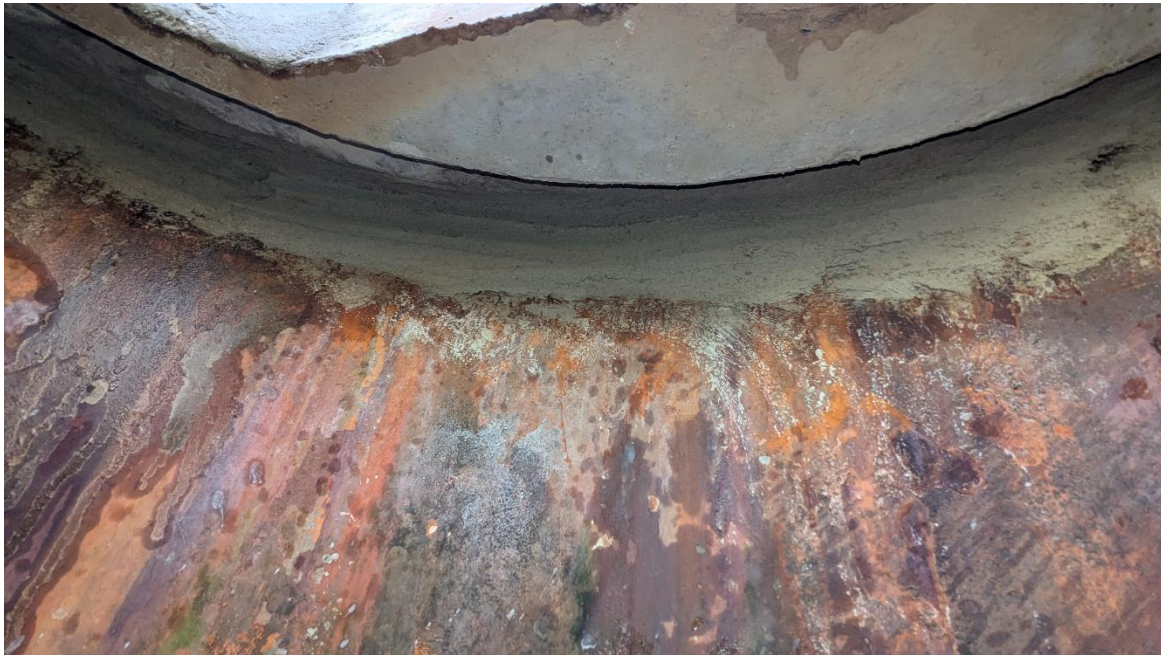
Figure 7 Image from inside structure where gap was repaired with waterproof mortar
