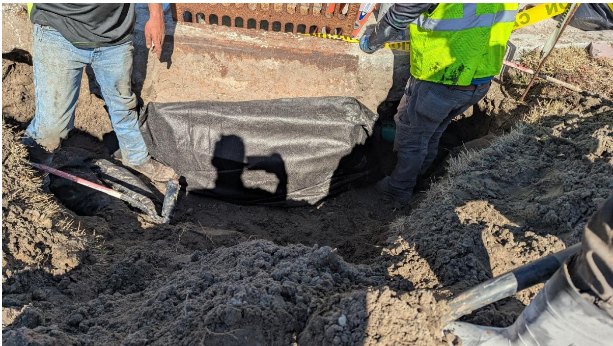
Figure 6 Wrapping repaired area in filter fabric prior to backfill
