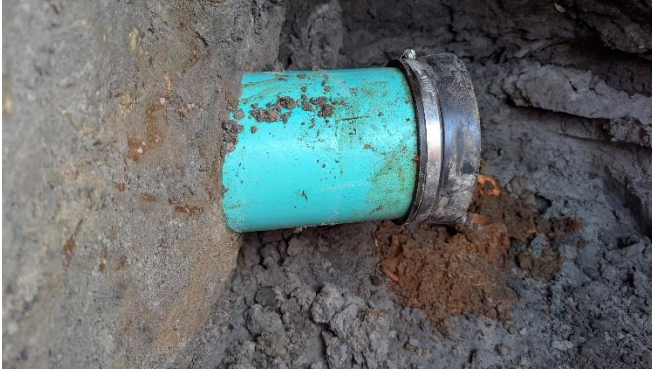
Figure 3 New solid cap added to underdrain stub on east side of structure. No damage present. Contractor wanted to put new cap to ensure proper seal.
