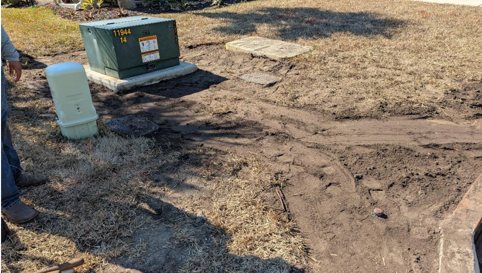
Figure 9 Completion of grading and compaction after FPL transformer was reset
