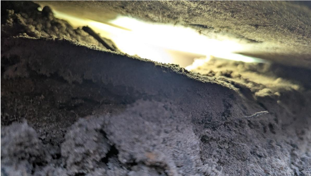
Figure 1 Photo taken from outside of structure showing gap through top section. Contractor is shining flashlight from inside of structure
