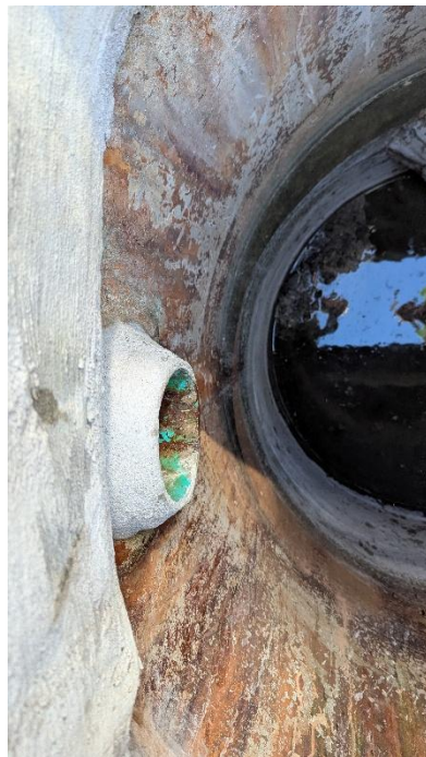
Figure 8 (Left) mud work around underdrain stub. Not required but performed by contractor for additional sealing. (Right) structure with wate and soil removed while plug was still in place. Note that pipe seen will normally be submerged as designed.
